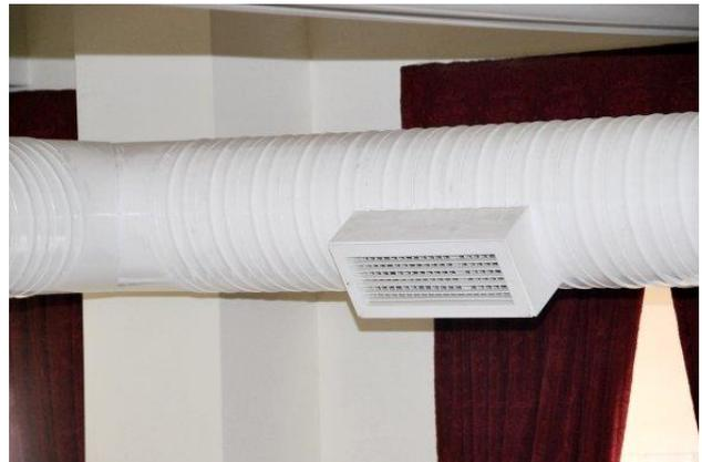
*The heat pump is plumbed into the grey pipes and electrics ... air is delivered everywhere, via standard ducting*
